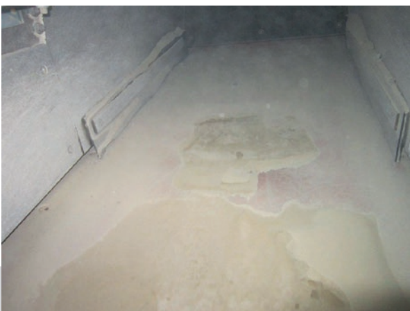
Ansicht 1 Conveyor chute with PUCEST ® lining, after 7 months of permanent load
