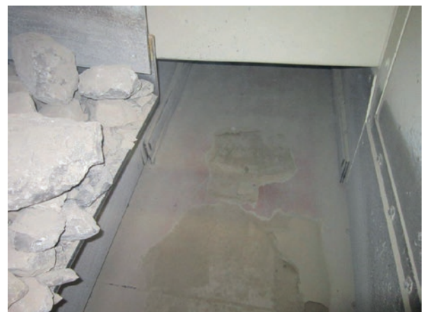
Ansicht 2 Conveyor chute with PUCEST ® lining, after 7 months of permanent load
