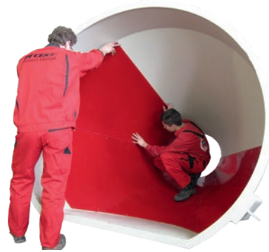
▲ The liner was fitted into the hopper.
